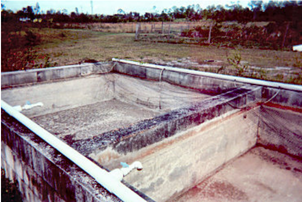
Empty concrete vats
